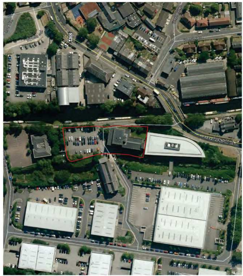
Existing Office Building Location
